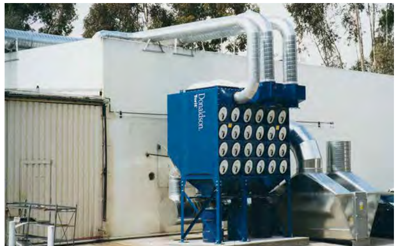
DFO on Metal Grinding 31,000 cfm (52,658 m 3 /h)
