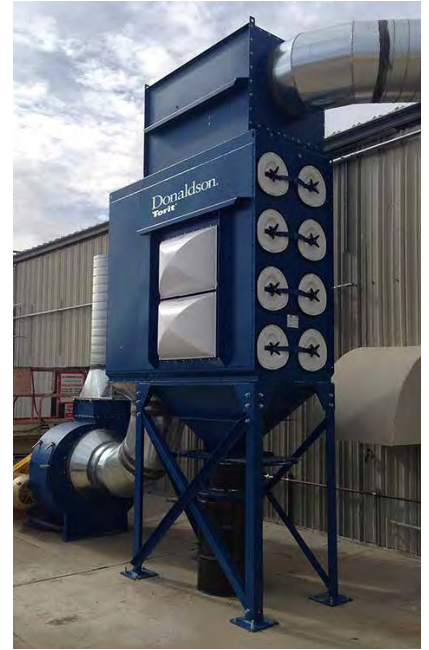
DFO on Plastics Routing 16,000 cfm (27,184 m 3 /h)
