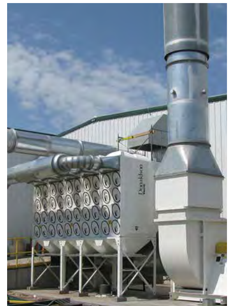
DFO on Corn Husking & Sorting 28,500 cfm (48,412 m 3 /h)
