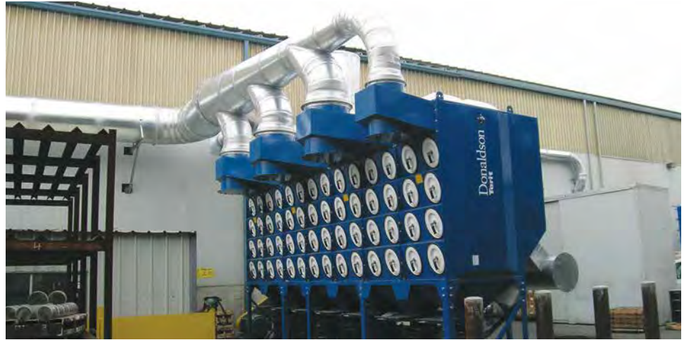
DFO on Grinding 74,000 cfm (125,700 m 3 /h)
