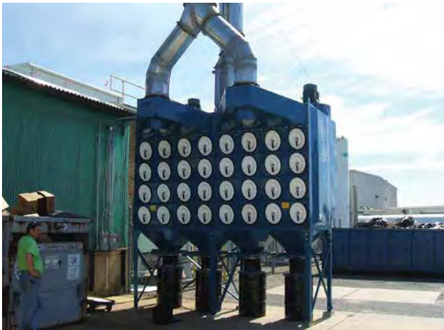
DFO on Thermal Spray 8,500 cfm (14,439 m 3 /h)
