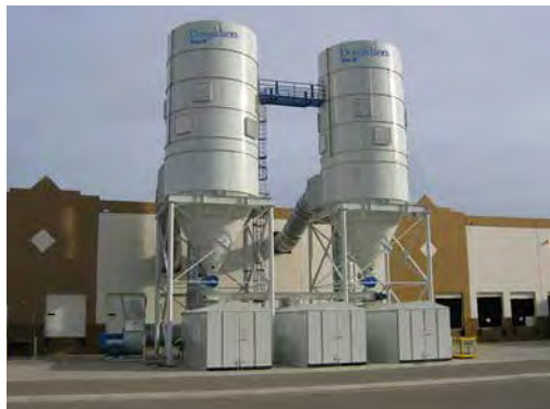
LP on Wood Dust 160,000 cfm (271,784 m 3 /h)
