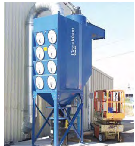
DFO on Plasma Cutting 5,000 cfm (8,493 m 3 /h)
