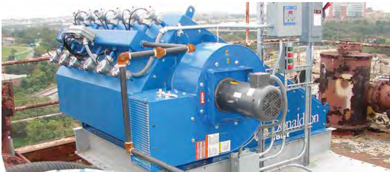
CPV - Multiple Cement Silos 4,800 cfm (8,154 m 3 /h)
