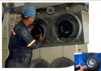
Note: If you perform filter maintenance service on a schedule vs. using service indicators, you may want to write the service date on the filter end cap.
