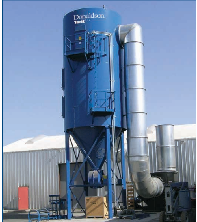
The Dura-Life bag filters in this Donaldson Torit RF Baghouse collector provide longer life and lower emissions at this Midwestern soybean processing plant.
