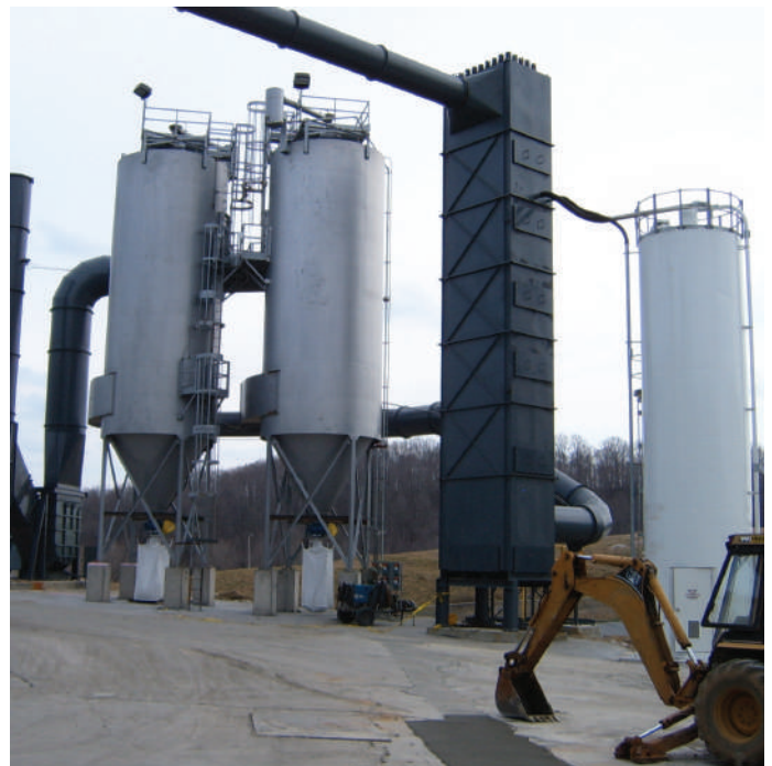
484RF - Two High Temperature Collectors on Secondary Aluminum Processing
