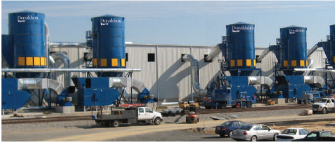
776RF at Wood Furniture Plant
