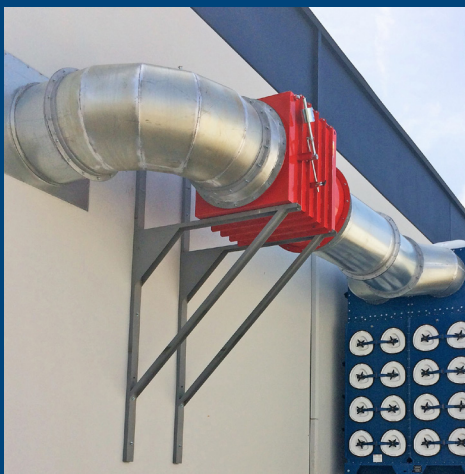
Flow-Actuated Isolation Valve
