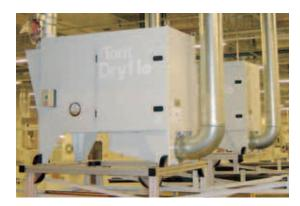
Both units are extremely efficient in operation and use Donaldson's operationally proven three-stage filtration system specifically engineered for mist collection. As the unit operates filtration cartridge efficiency increases.
